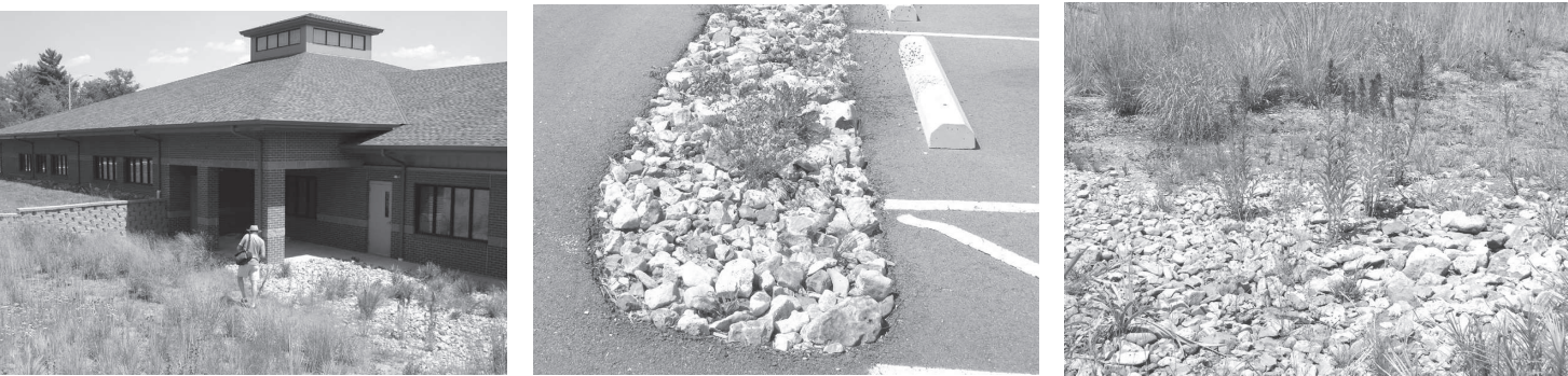
Left: Water flows off roof and into bioswale. Middle: Water runoff from parking lot enters bioswale. Right: Rain garden basin with wetland species and river gravel.
