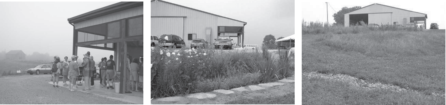
Left: Downspouts on building flow underground to rain garden. Middle: Rain garden with building in background. Right: Rain garden overflows through rock spillway to lower pond.
