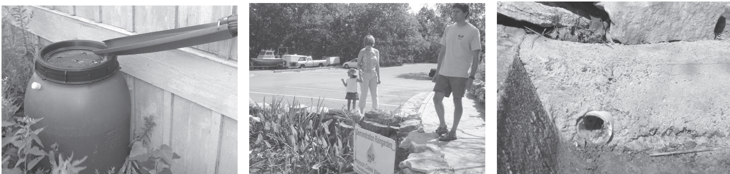
Left: Rain water enters rain barrel from downspout. Rain barrel overflows into basin. Middle: Rain garden basin with pickerel weed. Right: Rain garden overflows into parking lot.
