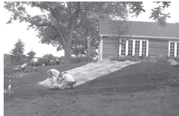
Above: Wood shavings erosion control mat shown interplanted with sedges.
